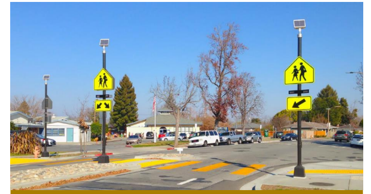
Rectangular Rapid Flashing Beacon (RRFB)
